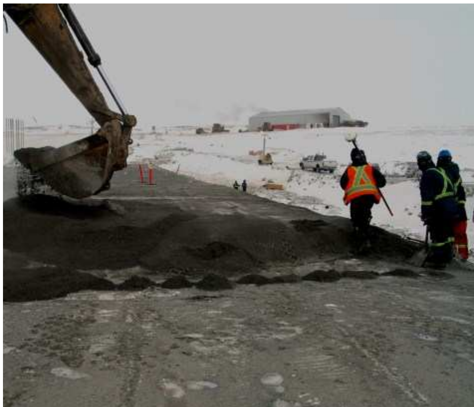
Photo 4: Placing ROQ. Thermistor installation in foreground
