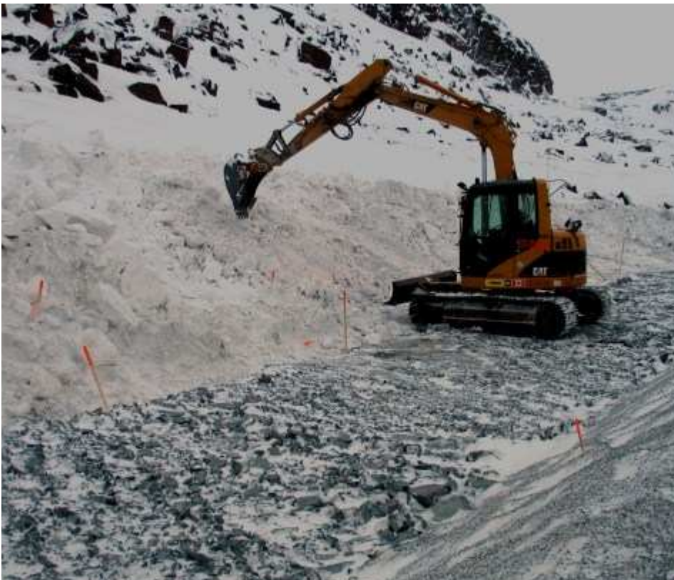
Photo 13: Small excavator pushing snow from back of trench
