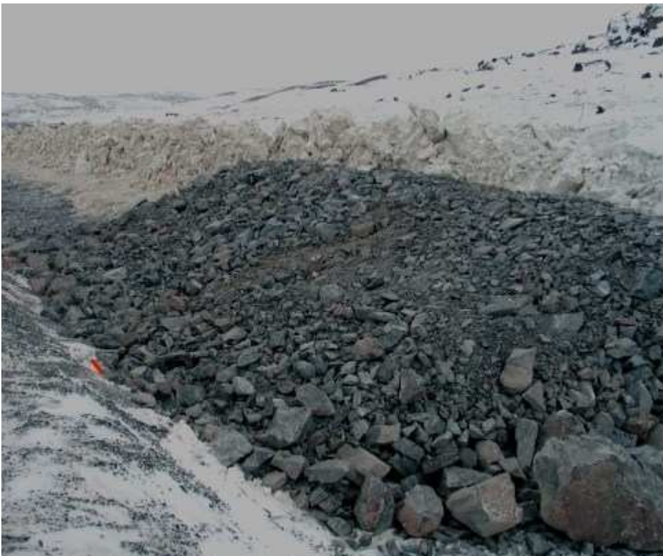
Photo 12: Start of second lift ROQ between Sta 3+95 and Sta 4+45
