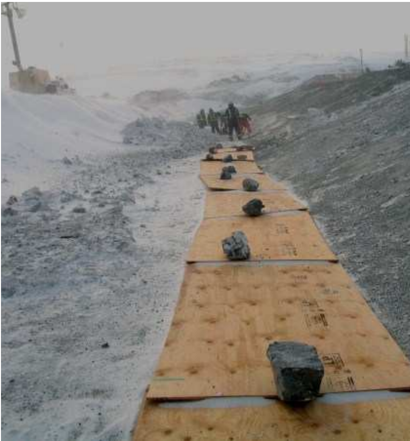
Photo 7: Plywood placed over cleaned GCL
