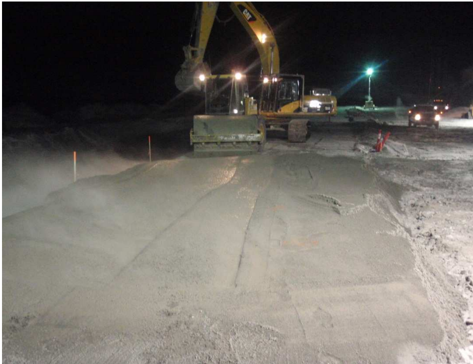
Photo 16: Packing completing static passes on FCM around station 1+40. Note that later / after vibrator compaction effort was also used.
