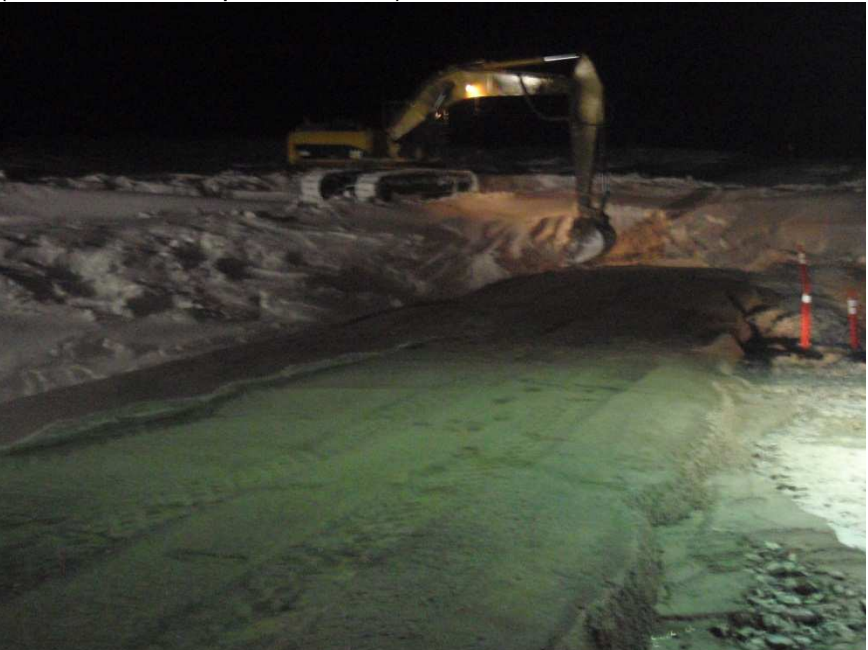
Photo 21: Excavator starting to remove snow from around S end of dam
