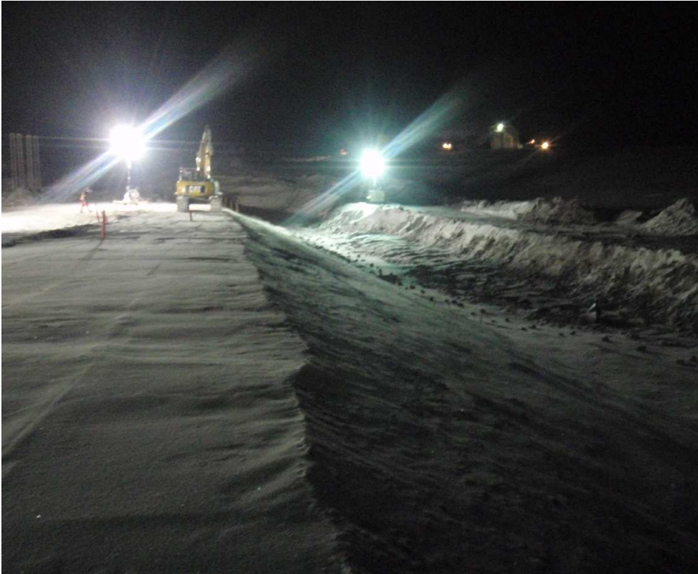
Photo 14: ~NE view down upstream crest of dam. Note the 330 in the background scraping down the areas where nightshift placement started.
