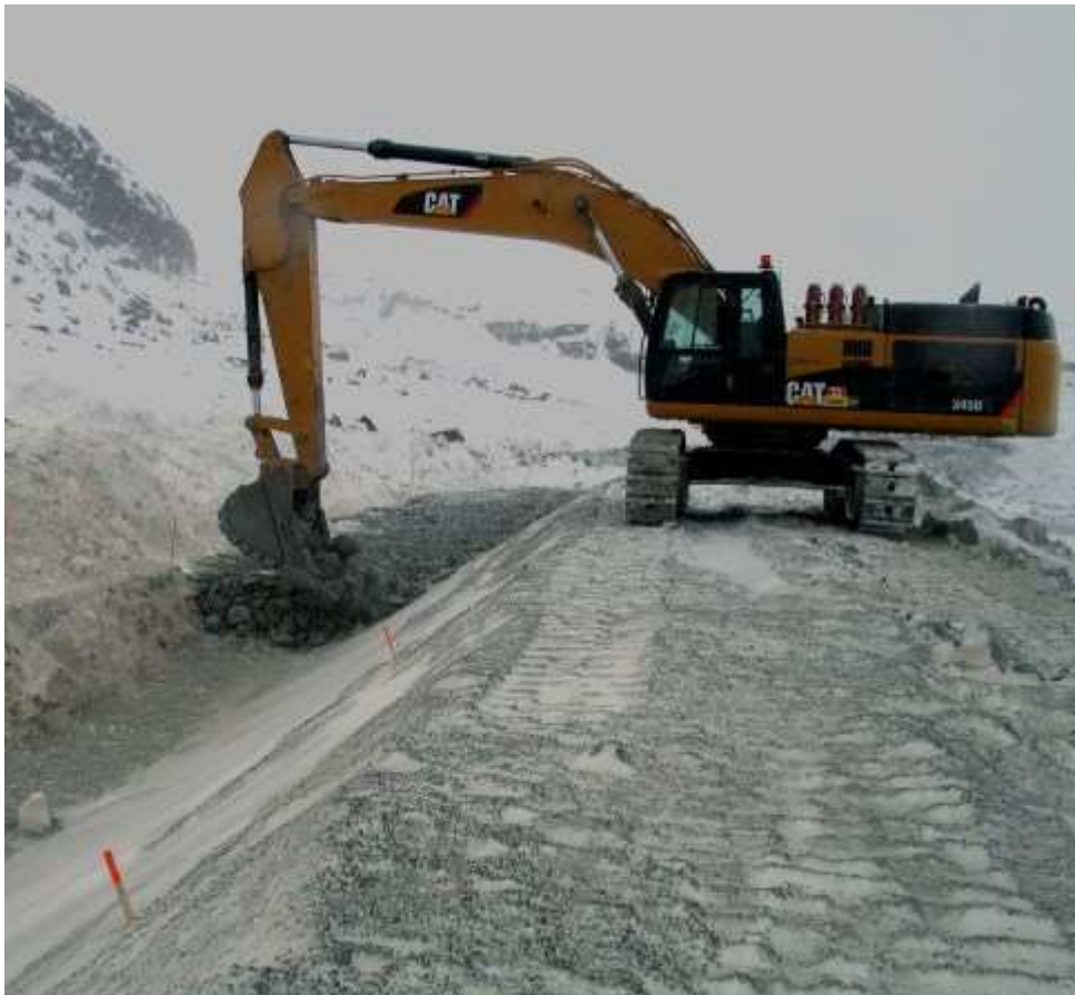
Photo 10: Excavator placing ROQ between Stn 5+35 and Stn 5+85
