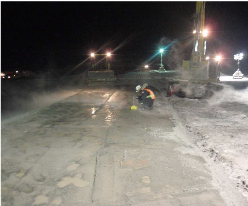
Photo 17: EBA testing FCM placement with nuke around station 1+40.
